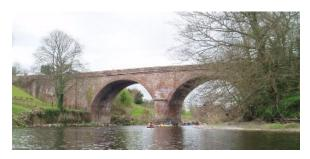
The new bridge was downstream of the previous bridge and much higher with a large embankment created on either bank to reduce the gradient of the road on each side.
